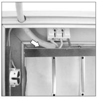
Connect the cable into the terminal block.
