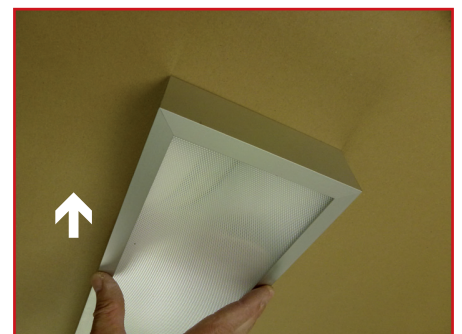
9. Abdeckung zuklappen / close and fix cover
