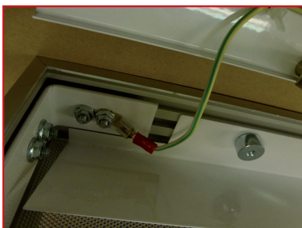
7. Erdkontakt anschliessen / connect earthing contact
