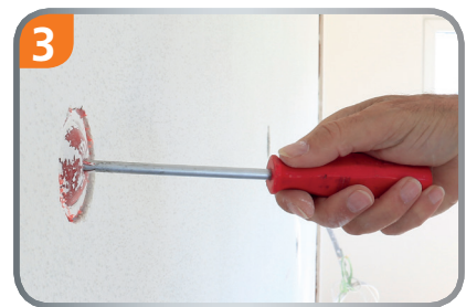
Finally, use a screwdriver to remove the plaster cover.
