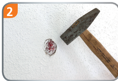
Slightly hit the plaster cover with a hammer.
