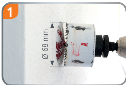
Mill with a bit \varnothing 68 mm around the plaster cover.
