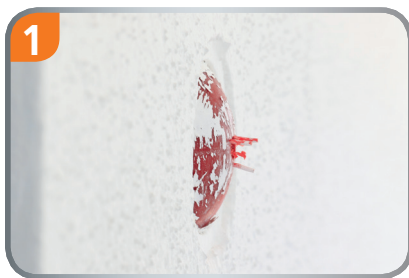
After plastering, the plaster cover protrudes.
