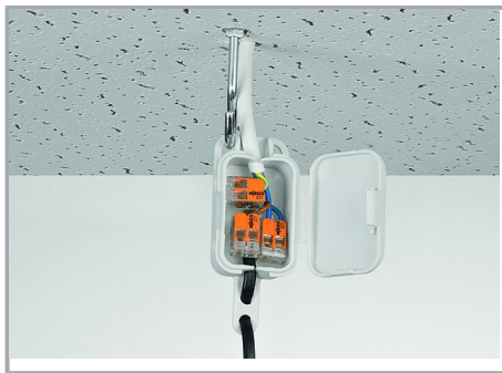
Pendant light connection in a suspended ceiling
