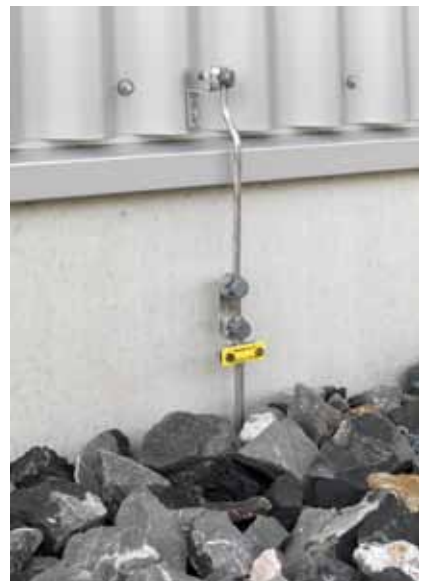
Separation point in an earthing system
