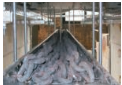
Steel chains as replacement weights
