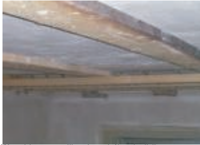
Wood beam ceiling in existing building
