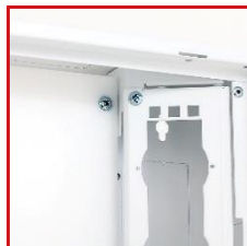
Empty opening for power socket
