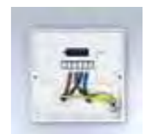
Large terminal compartment
