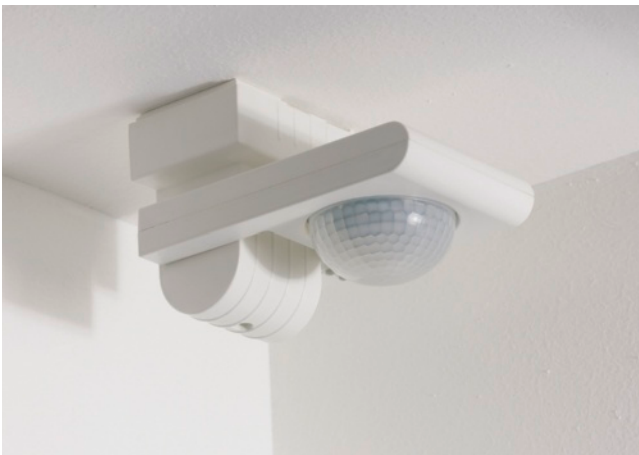
Mounting of motion detector on the ceiling
