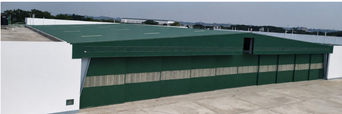
Fig. 4 Aircraft hangar shed after completion
