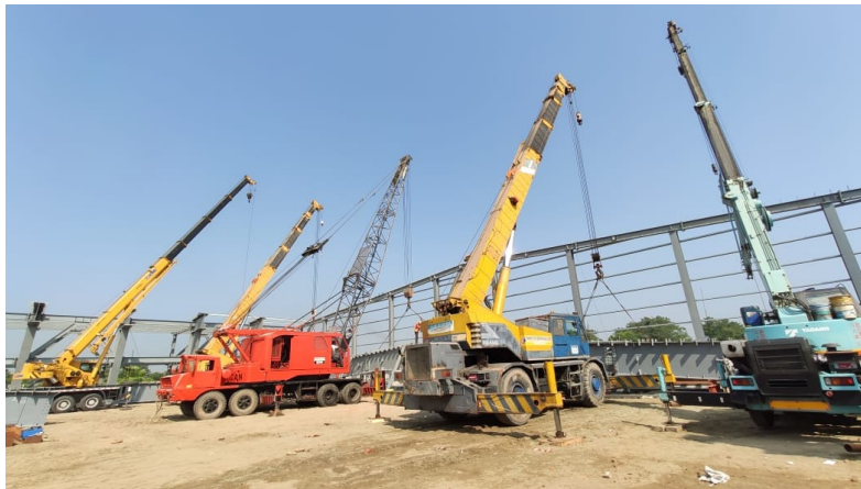
Fig. 20 Cranes used in lifting operation
