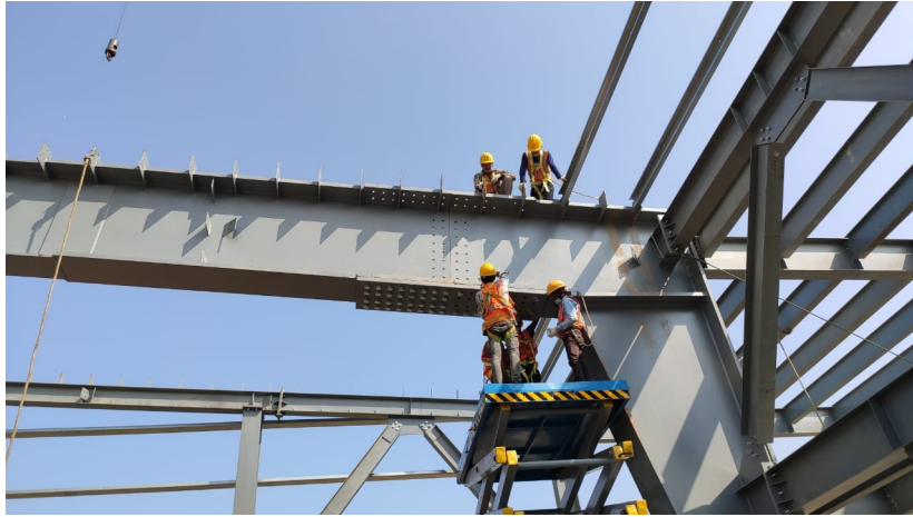
Fig. 19 Installation of the connection between the rafter and the L-shaped column
