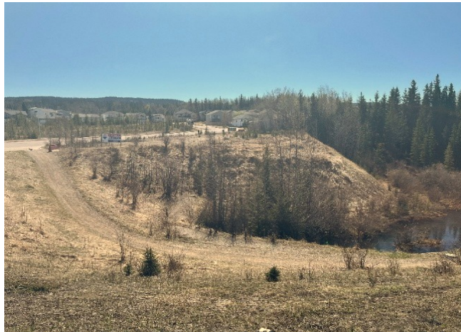
Fig. 4. Rear site condition showing slope transition toward the ravine and adjacent low-lying area.
