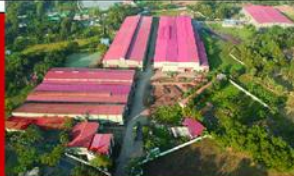
STEELMARK BUILDINGS LTD
