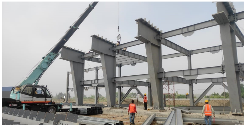
Fig. 18 Erection of office buildings and L-shaped columns of the shed
