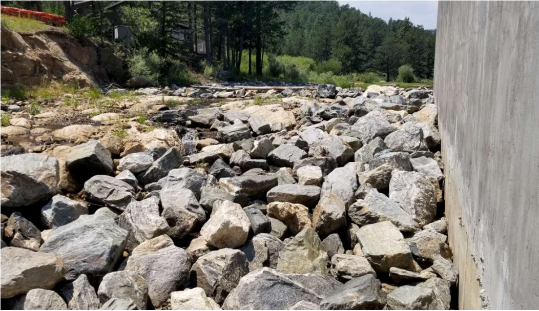
Typical photo of the emergency spillway crest and downstream channel.
