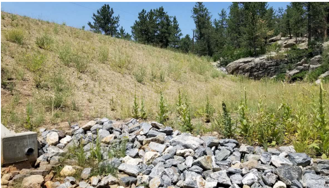
Photo along the downstream slope. Note sparse vegetation growth.
