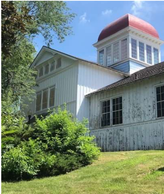
Pioneer Hall – West Entrance upgrade, new roofing
