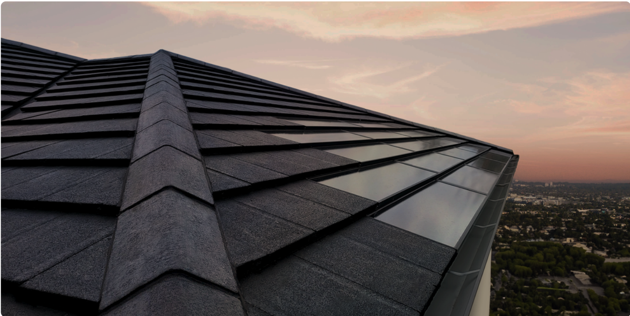
Image: Volt Solar Tile (Lodge) installation, Eltham, Victoria [Background edited for illustrative purposes]
