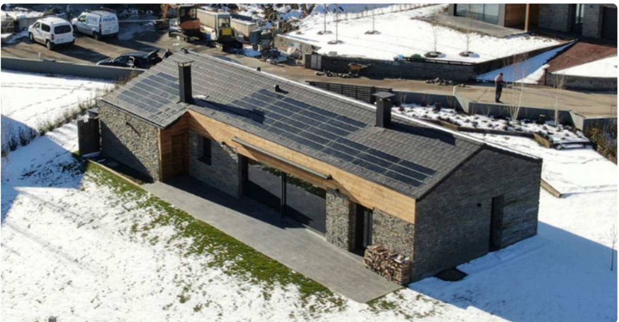
Image: Volt Solar Tile installation, Cerdanya, France
