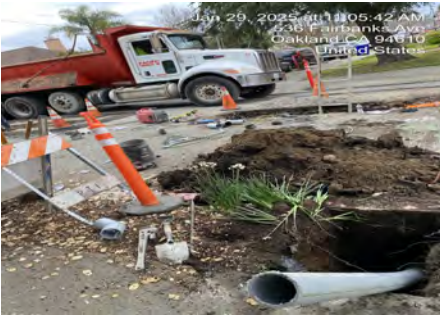
Sanitary Sewer Rehabilitation - Sub-Basin 84-004
