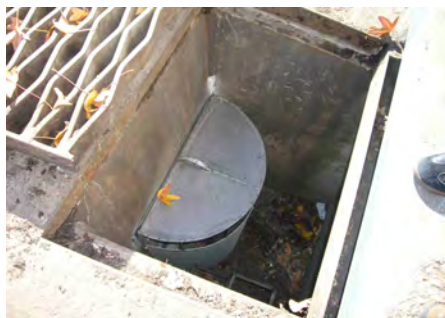
Citywide Storm Drainage Replacement
