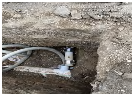
Sanitary Sewer Rehabilitation - Sub-Basin 81-002
