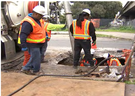
Emergency Roadway Reconstruction
