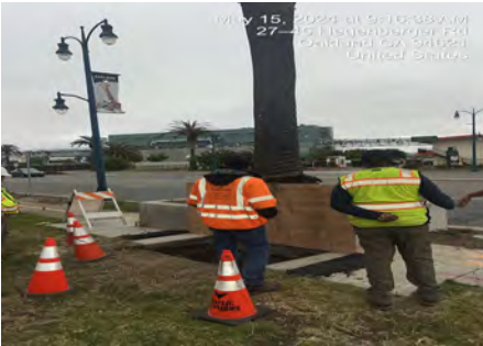
Sanitary Sewer Rehabilitation - Sub-Basin 62-02
