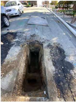
Sanitary Sewer Rehabilitation - Sub-Basin 85-231
