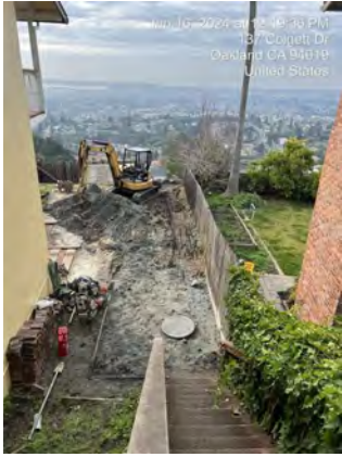
Sanitary Sewer Rehabilitation - Sub-Basin 85-102
