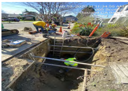
Sanitary Sewer Rehabilitation - Sub-Basin 81-001
