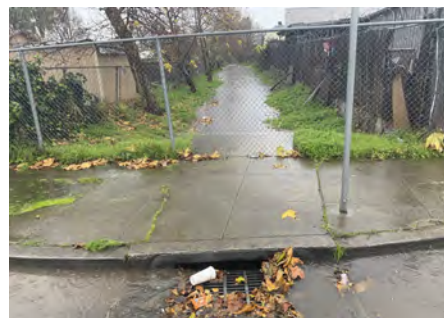
Empire Road Storm Drain Improvement
