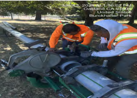
Sanitary Sewer Rehabilitation - Sub-Basin 83-201
