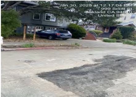
Sanitary Sewer Rehabilitation - Sub-Basin 84-101
