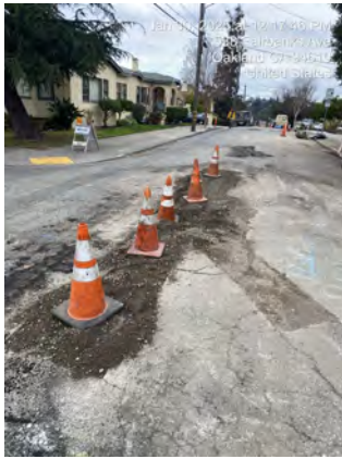
Sanitary Sewer Rehabilitation - Sub-Basin 85-211
