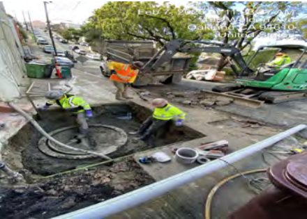
Sanitary Sewer Rehabilitation - Sub-Basin 56-02
