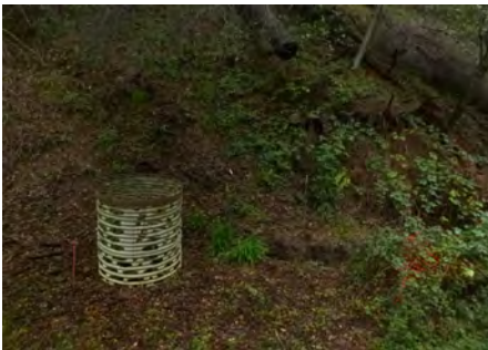
Beaconsfield Canyon Storm Drain Inlet Replacement
