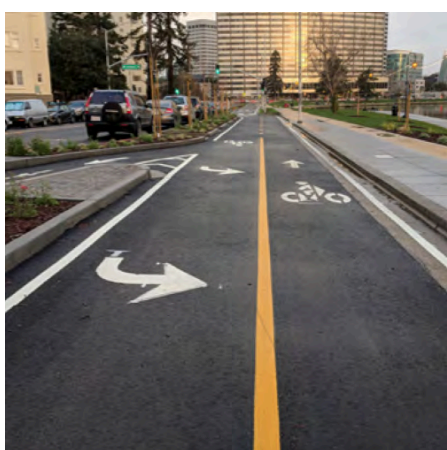
Lakeside Green Street
