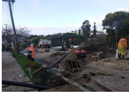
Hotspot Sewer Repair
