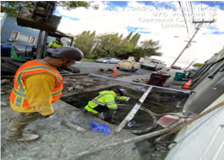
Sanitary Sewer Rehabilitation - Sub-Basin 60-03/17
