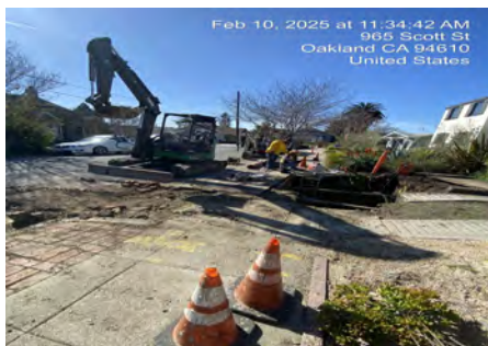
Sanitary Sewer Rehabilitation - Sub-Basin 80-001
