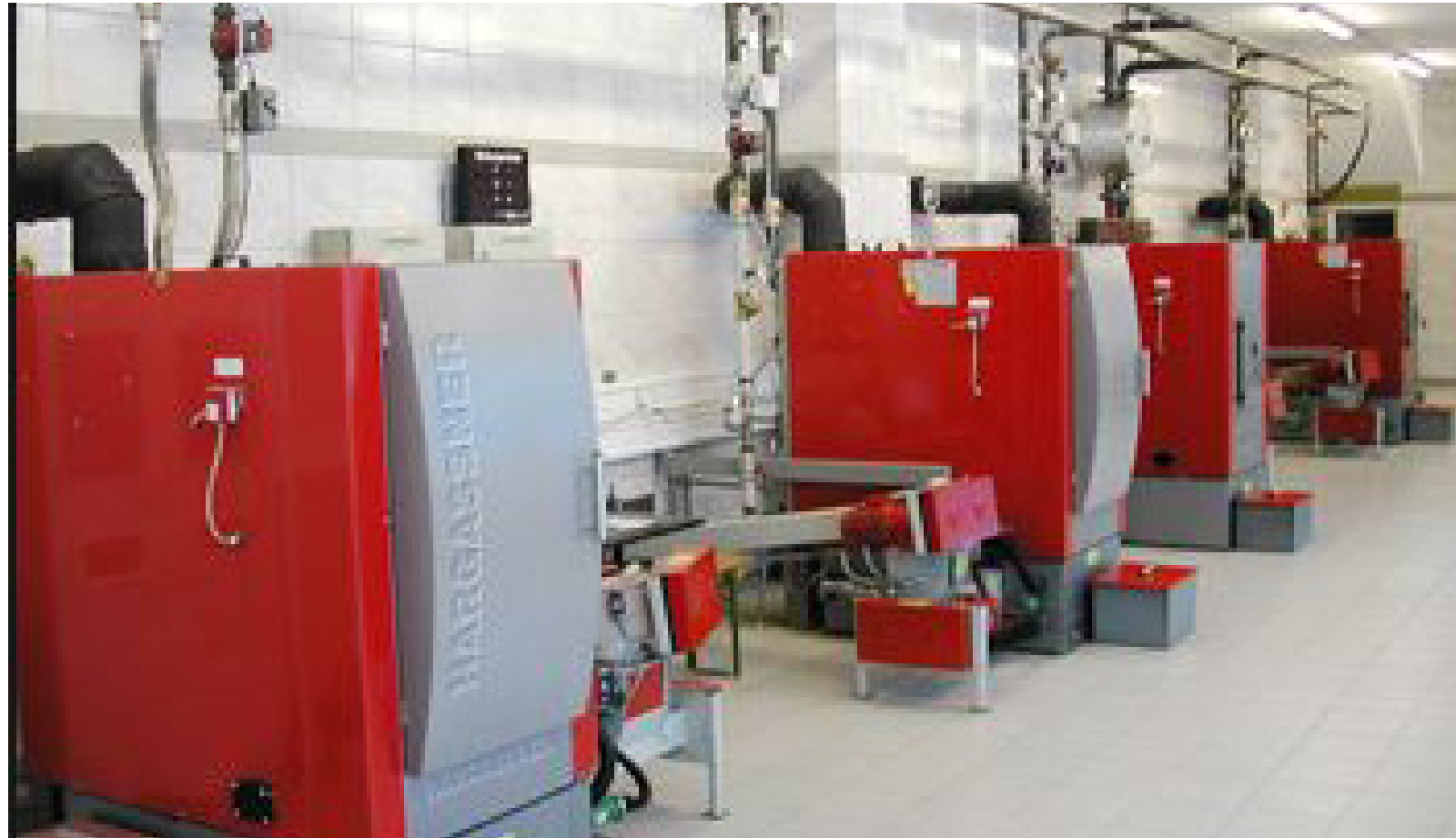
3: Hargassner Wood Gasification Boiler Fuelled by wilding conifer sourced woodchips (Made in Austria)
