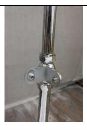
With one person holding and supporting the back glass, use the Allen key to tighten the glass to the corner connector.
