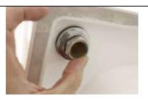
Slip both the nut and the brass compression washer from Part #004 over the post.
