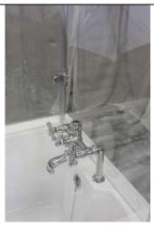
There are two sections to the shower riser. The top part has the L shaped showerhead holder and the bottom part is straight with one plain and one threaded end.
