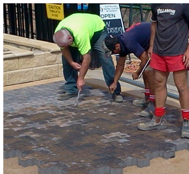
Spacing the pavers to keep straight lines.
