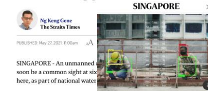
SINGAPORE - An unmanned soon be a common sight at six here, as part of national water HDB and A*Star to study using drones and robots to enhance construction site safety
