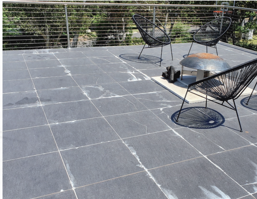
PHOTOGRAPH 3: This image shows extensive polymer leeching which began to take place early after completion. There was rain on the installation and the average temperatures in the installation period range from a high of 18 degrees Celsius and average low is nine degrees Celsius.
