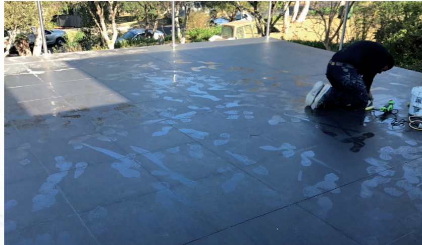
PHOTOGRAPH 7: This image shows adhesive on tiles in various states of final curing. The tile bonded around the edges strongly, then less well towards the centre where prolonged moisture content and slow setting has retarded the outcome. Poor trowel method has exacerbated this problem.
