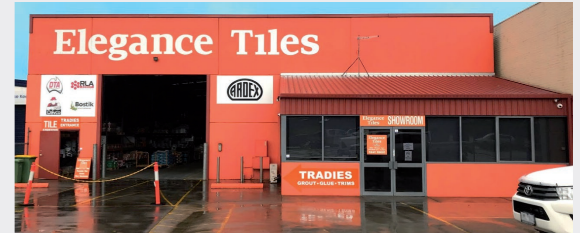
A view outside the Elegance Tiles Pakenham store
