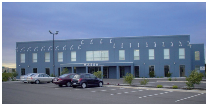
The purpose-built Massa Imports facility in Laverton North (VIC). Massimo and his staff moved into it in 2006.
