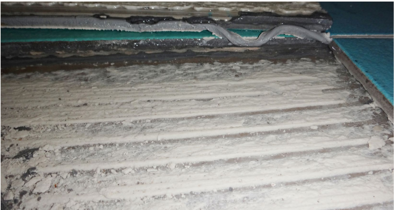
FIGURE 6. Here, 90% plus adhesive coverage did not prevent delamination. The shearing of the adhesive layer regularly leaves little adhesive at one edge and a proud rib on the opposite edge, again like waves coming into a beach.
