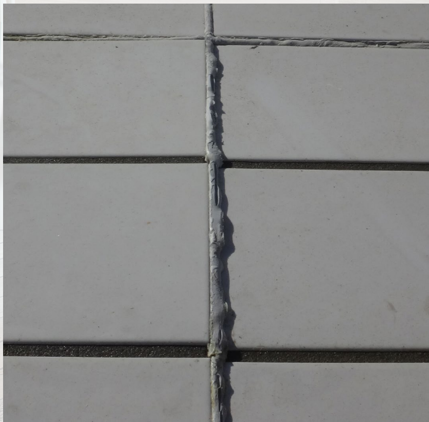
FIGURE 2. The intermediate movement joint at this location had been completely compressed and the sealant exuded. This shows shrinkage of the underlying concrete slab has occurred after the tiles were laid, as the underwater thermal conditions were relatively stable.
