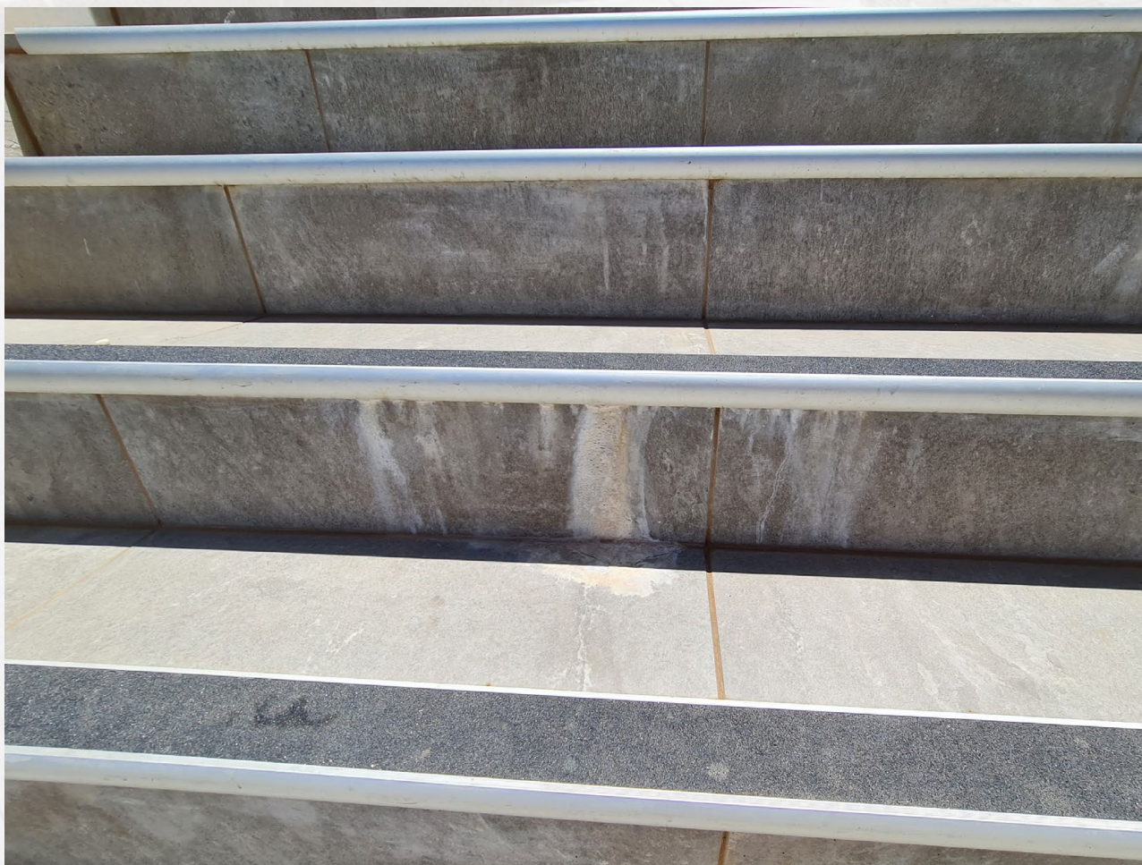
Efflorescence leeching from steps leading up to a pool concourse.
