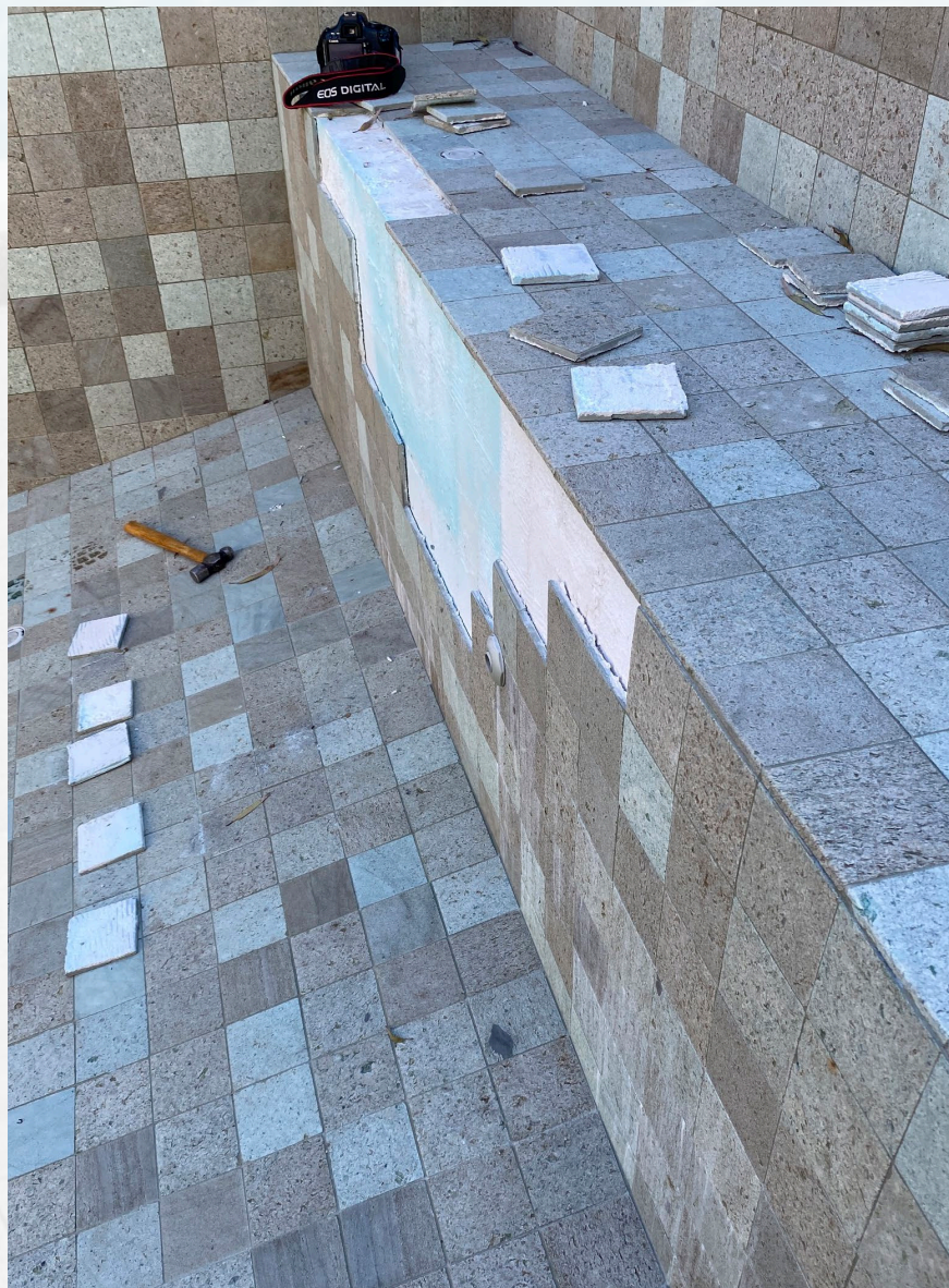
Adhesive bond failure due to omitting movement joints in the tiling installation
