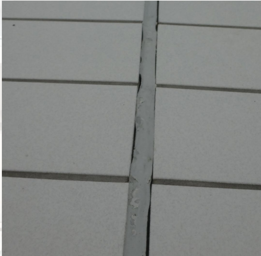
FIGURE 1. Shrinkage of the independent slabs at this construction joint has stretched the elastic joint so it detaches from the sides, strongly indicating that the concrete has shrunk after the tiles and sealant were installed.
