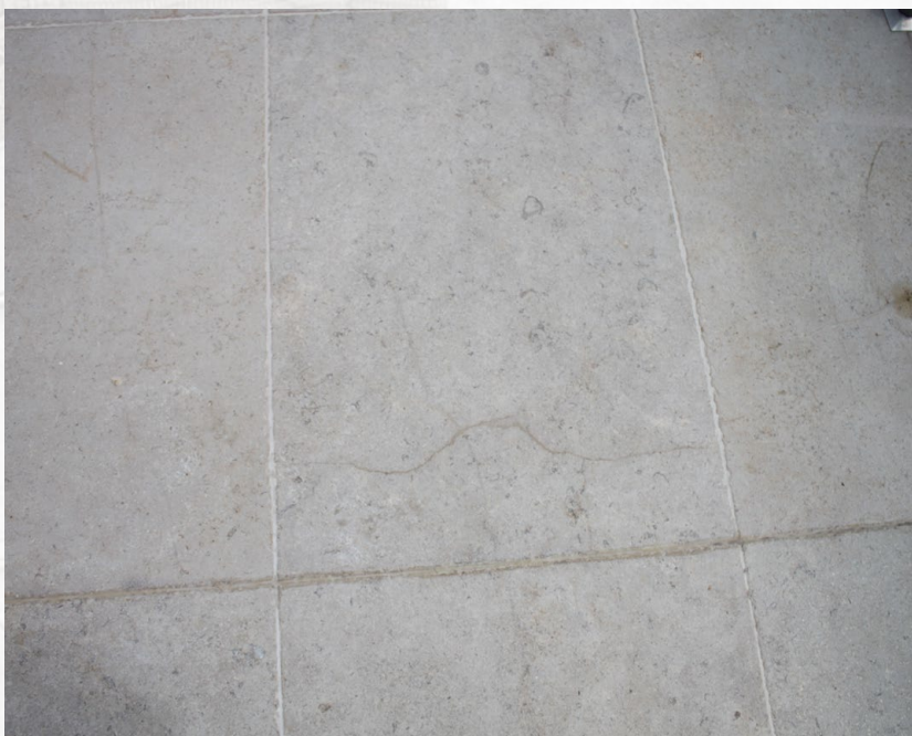
Cracking due to moisture exiting the face of stone tiles
