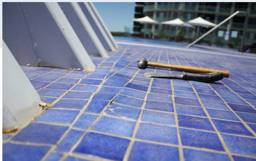
Tiles delaminating or 'tenting' due to lack of expansion joints.
