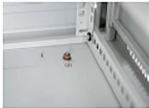
• Earthing screw inside
