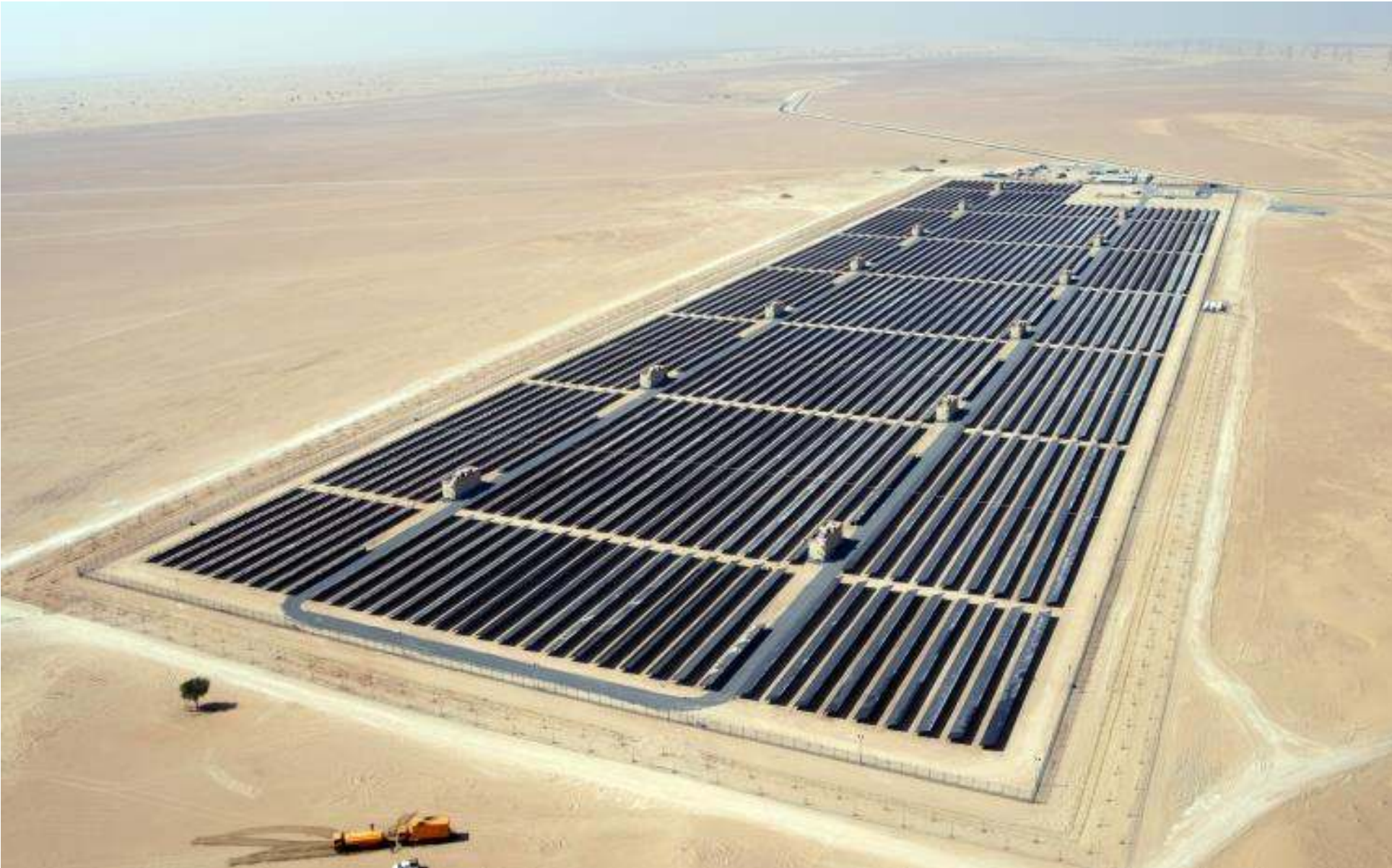
Phase 1 (200 MW) of the Mohammed bin Rashid Al Maktoum Solar Park. Source: First Solar
