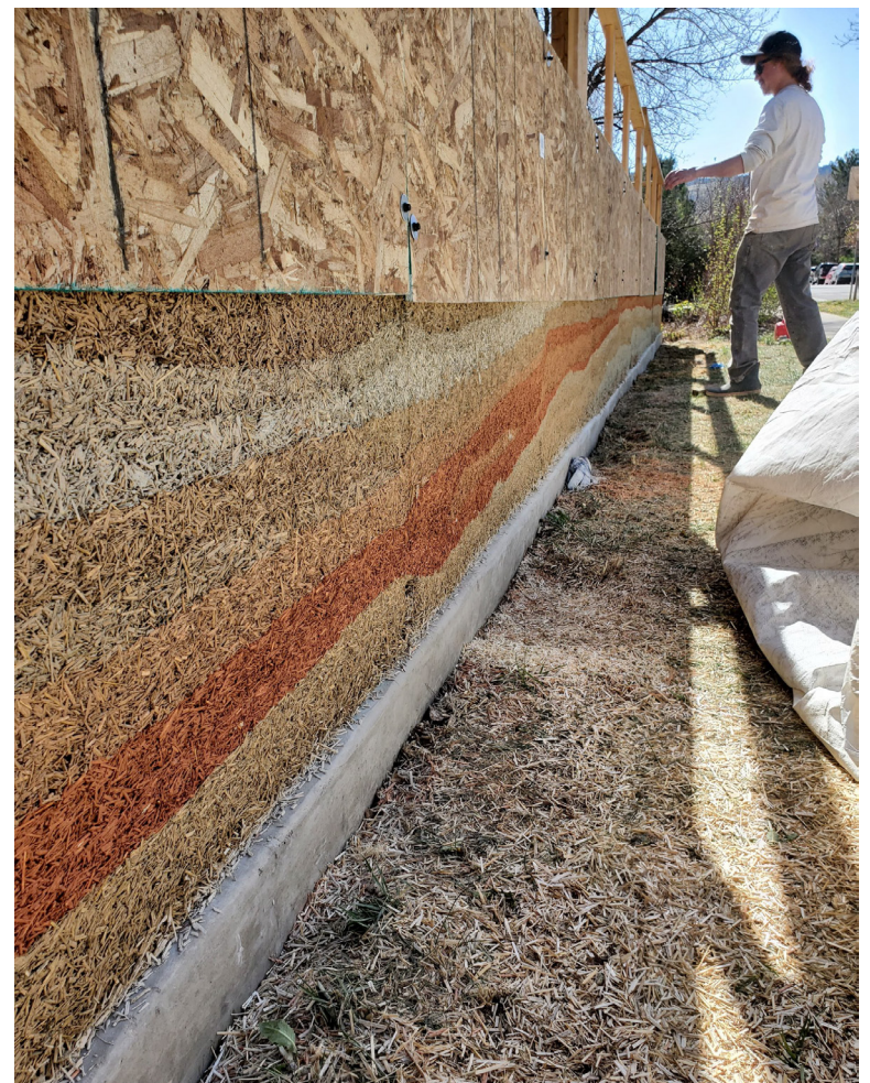
Hempcrete being deployed at the human scale, https://natural-building-alliance.org/hempcrete/
