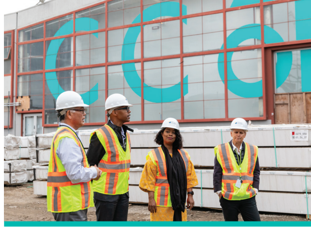
President Howse takes a hard-hat tour of the campus expansion, set to be completed by the time students return this fall.
