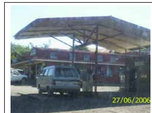
Figure 6: Plans are in place to upgrade standards and conditions of existing and new service stations as part of petroleum licence requirements.
