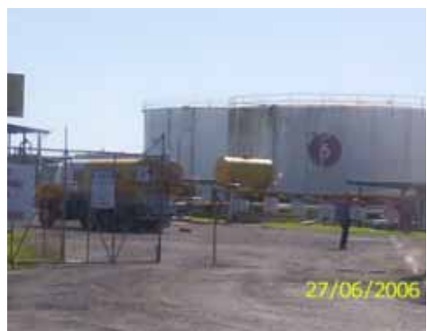
Figure 15: Petroleum storage facilities must adhere to national and international safety and quality standards.
