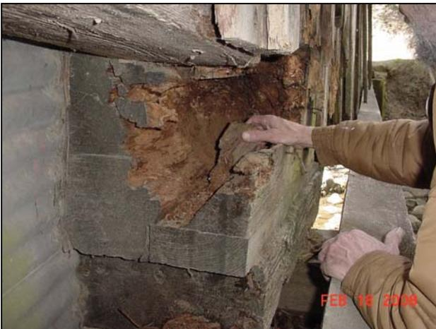
Decayed truss beam - I noticed the whole bridge span has a sag which does not show in pictures from the '70's.
