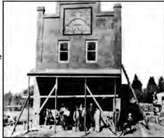
"The Mayo" Being Rebuilt, 1908 Courtesy of the Leland Pauley Collection
