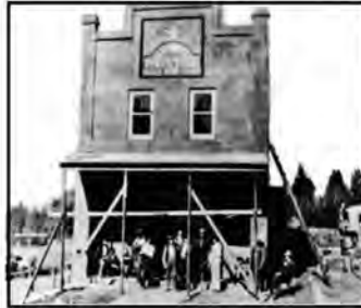
Rebuilding of "The Mayo," 1908 Courtesy of the Leland Pauley Collection
