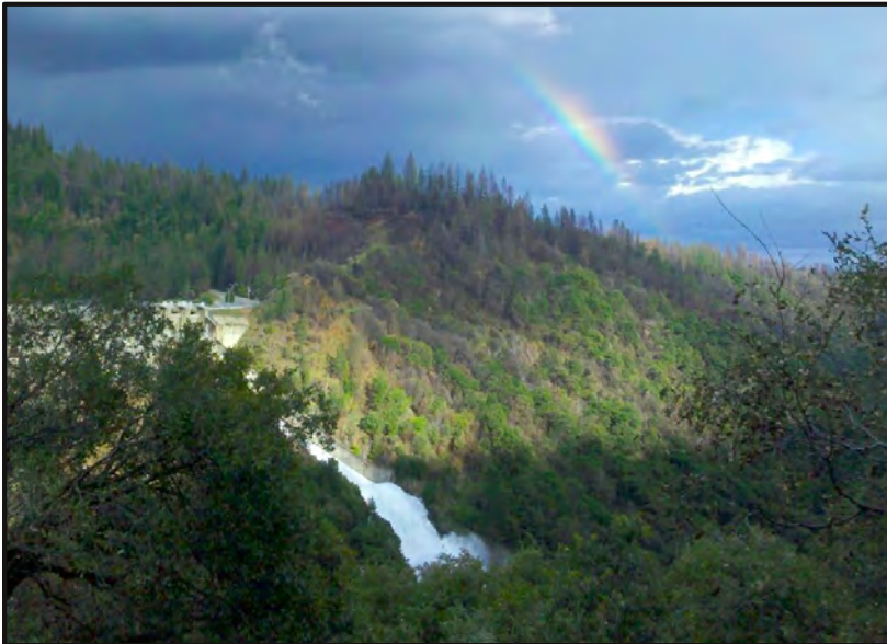
Bullards Bar spillway and rainbow!
