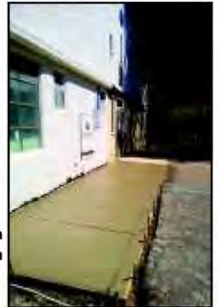
Cement poured for a new front porch
