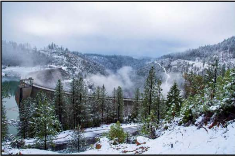
Early Snowfall Over Bullards Bar Dam
