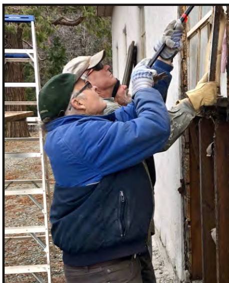
Above: Keith, Bob, and Norm pry out the kitchen window.
