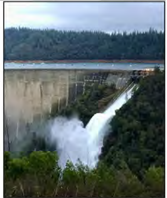
Water release at Bullards Bar Photo by Janie Kesselman
