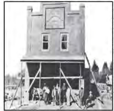
The Mayo construction crew, 1908
