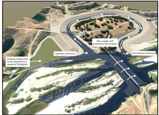
A rendering of the Nature-like Fishway around Daguerre Point Dam on the south side of the lower Yuba River. This view shows the existing intake area, which will be restored to a seasonal floodplain and the new intake and protective fish screens on the upstream entrance of the fishway. The outer wall of the fishway is designed to be flood resilient. The bridge over the fishway is an access bridge for operations and maintenance.
