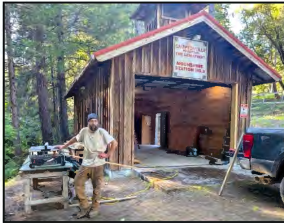
Angus working on the fire station
