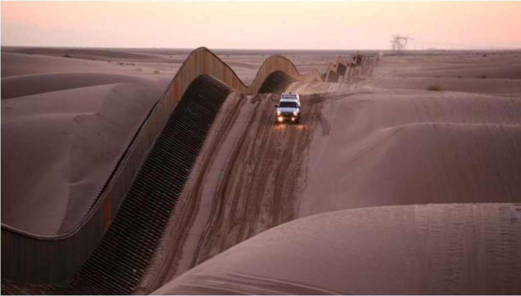
U.S. Border Patrol at Algodones Sand Dunes, California. The fence on the U.S.-Mexican border is a special construction of narrow, 15-foot-tall elements that are movable vertically. This way, they can be lifted on top of the ever shifting sand dunes. United States Department of Homeland Security
