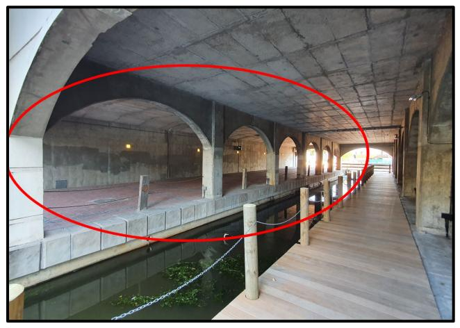
The underpass comprises a wide brick paved pedestrian walkway flanked by a concrete bridge abutment with four panels on the one side and seven pillars/six arches and the Grand Canal on the other side. The dimensions are approximately as depicted in the images below. The face surface is concrete and will require appropriate surface preparation.
