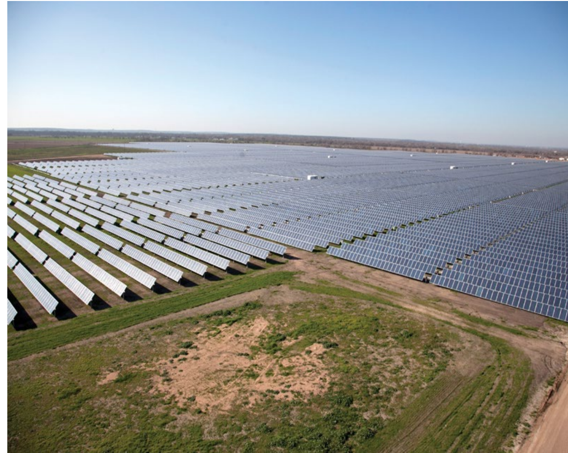
Webberville Solar Field (TX)
