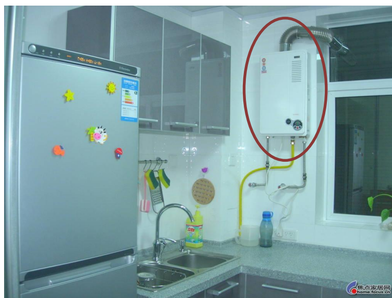
Figure 67: Example of gas instantaneous water heater installation 91
