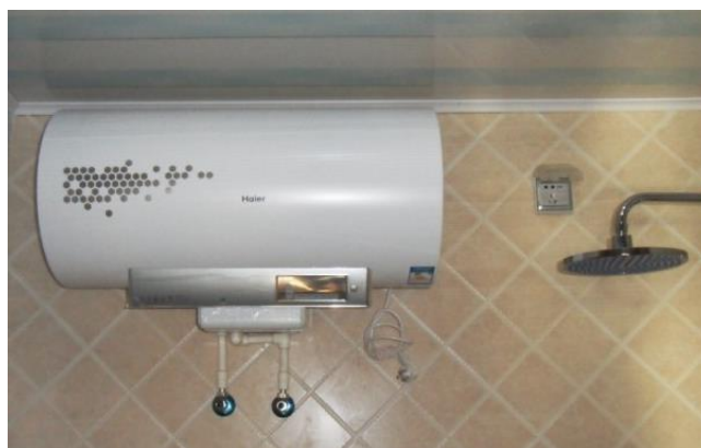
Figure 65: Example of electrical storage water heater installation 89
