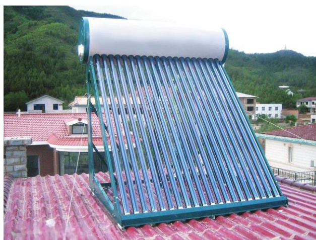
Figure 68: Example of solar water heater installation
