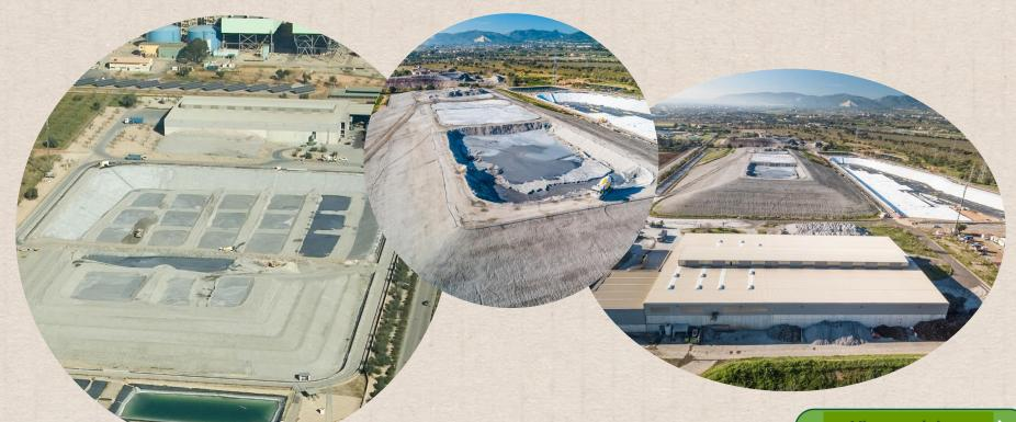
Our **secure landfill** receives the gas cleaning waste generated during the energy recovery process. This waste is previously stabilised by mixing it with cement and water.
