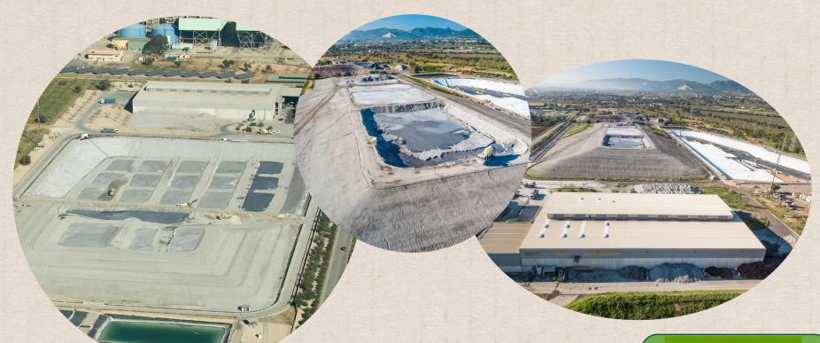
Our **secure landfill** receives the gas cleaning waste generated during the energy recovery process. This waste is previously stabilised by mixing it with cement and water.
