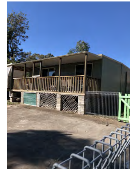
2. Exterior of building is unwelcoming
