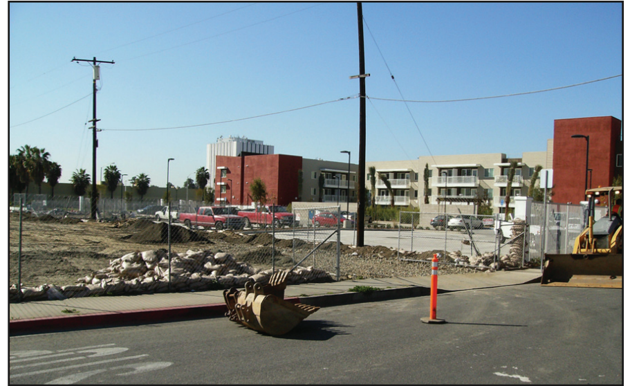
View 2: From the east side of E. Arbutus Street looking southeast at the Project Site.
