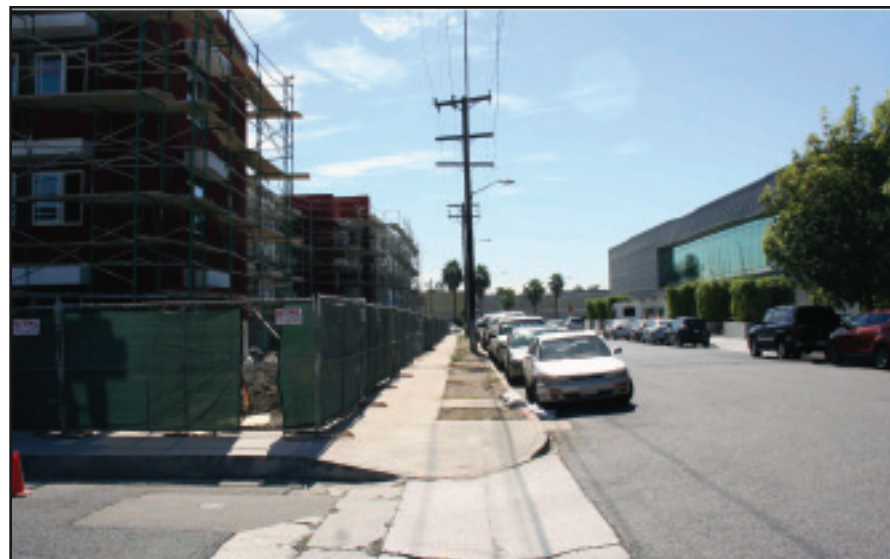
View 14: From the north side of the intersection of N. Tamarinda Avenue and E. Arbutus Street looking south.
