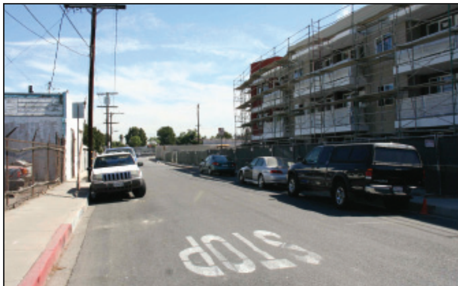
View 13: From the west side of the intersection of N. Tamarinda Avenue and E. Arbutus Street looking east.
