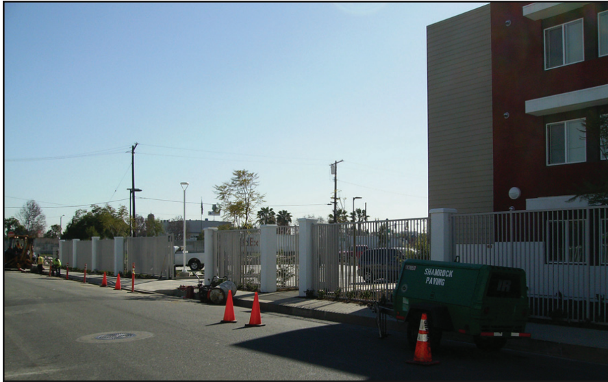
View 1: From the east side of E. Arbutus Street looking southeast at the Project Site.
