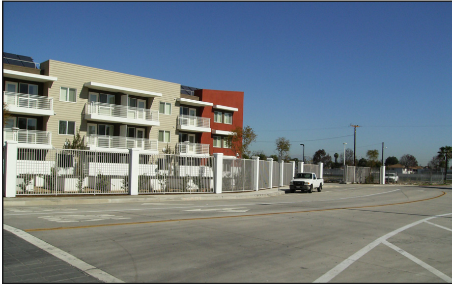
View 9: From the south side of E. Carson Place looking northeast.
