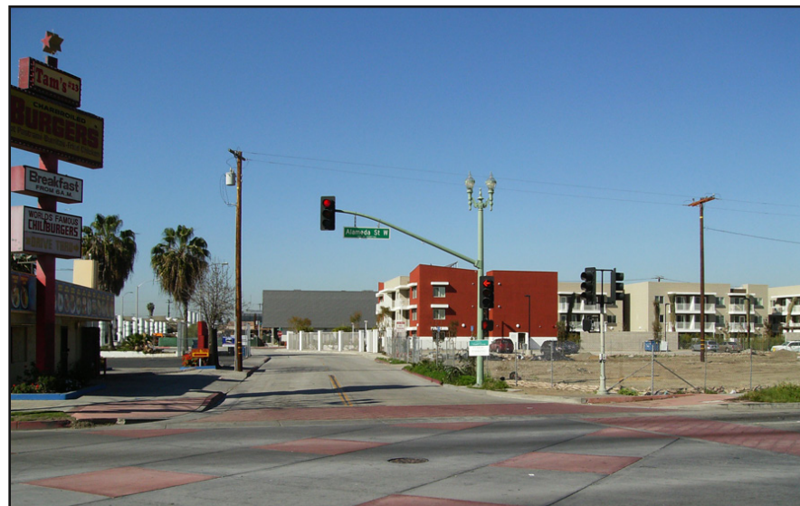
View 6: From the northeast corner of N. Alameda Street and E. Carson Place looking west at the Project Site.
