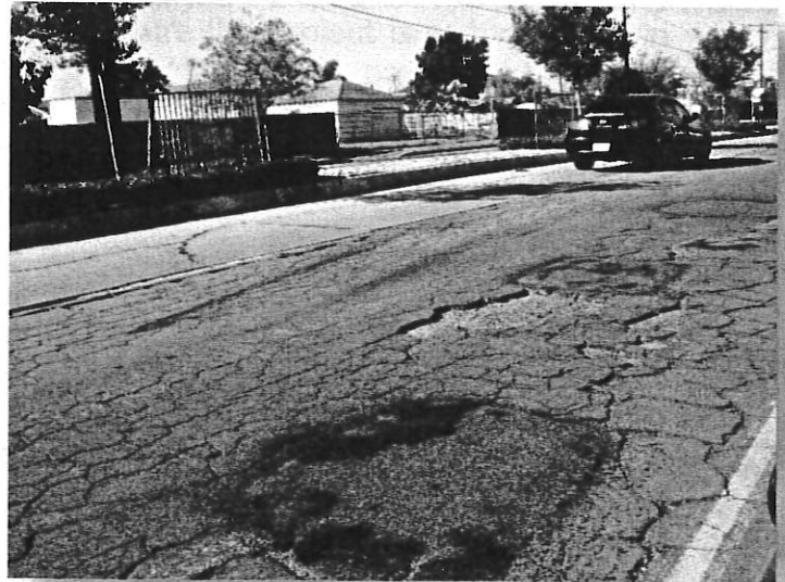
Figure 5: Current Condition of Central Avenue along Project Limits
