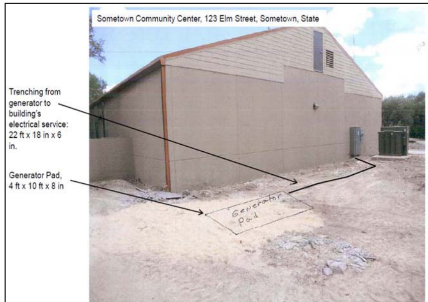
Figure 4. Ground-level photograph showing proposed ground disturbance area.
