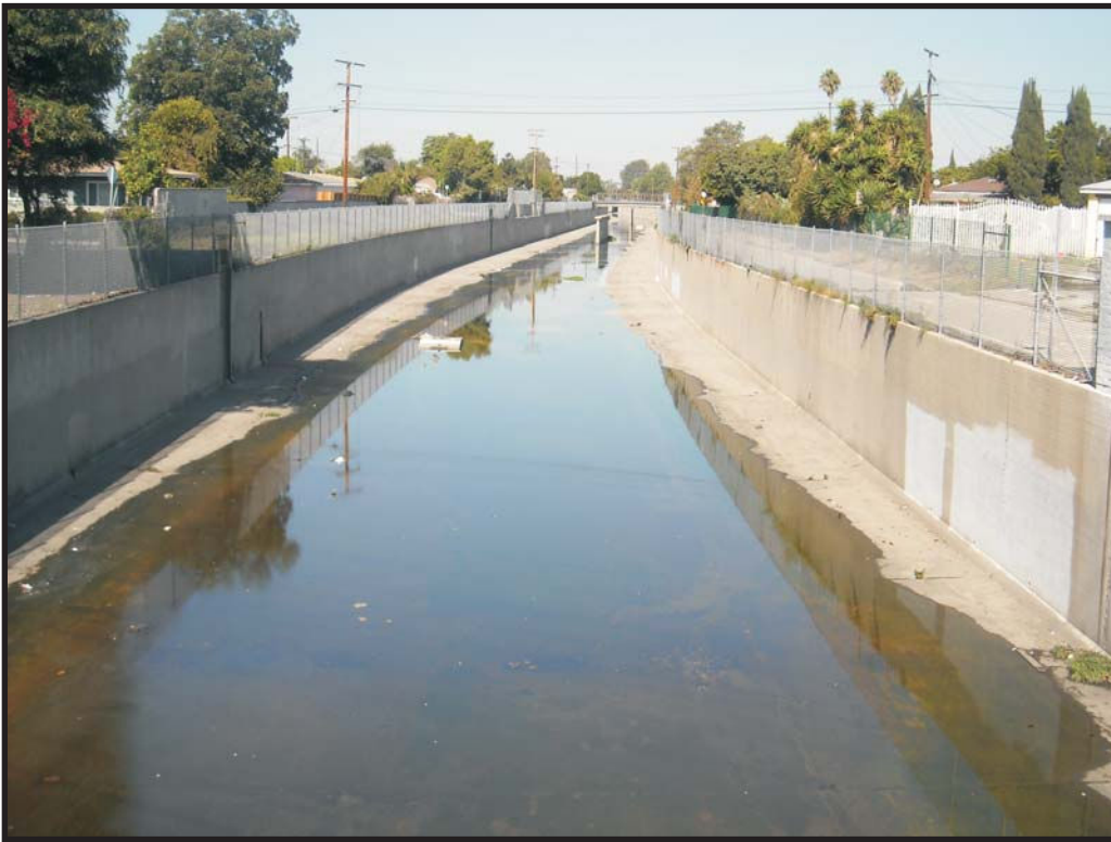
View of existing Compton Creek conditions at Greenleaf Boulevard looking north.
