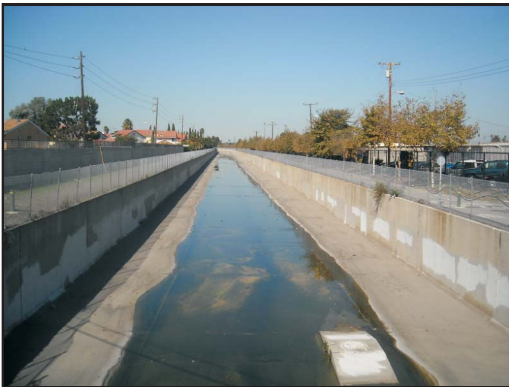
View of typical channelized segment of Compton Creek.
