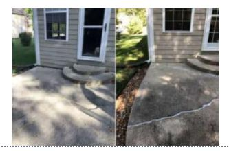
These photos were taken before and after an Acculevel crew slabjacked the porch back into position. You'll notice the gap between the siding and porch is closed, and sealant has been applied to repair the crack.
