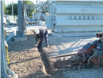
Dike installation for large equipment.
