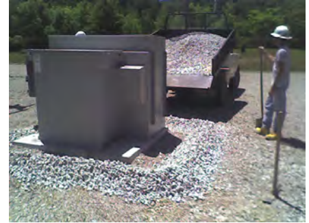
Pad mount for smaller containment.
